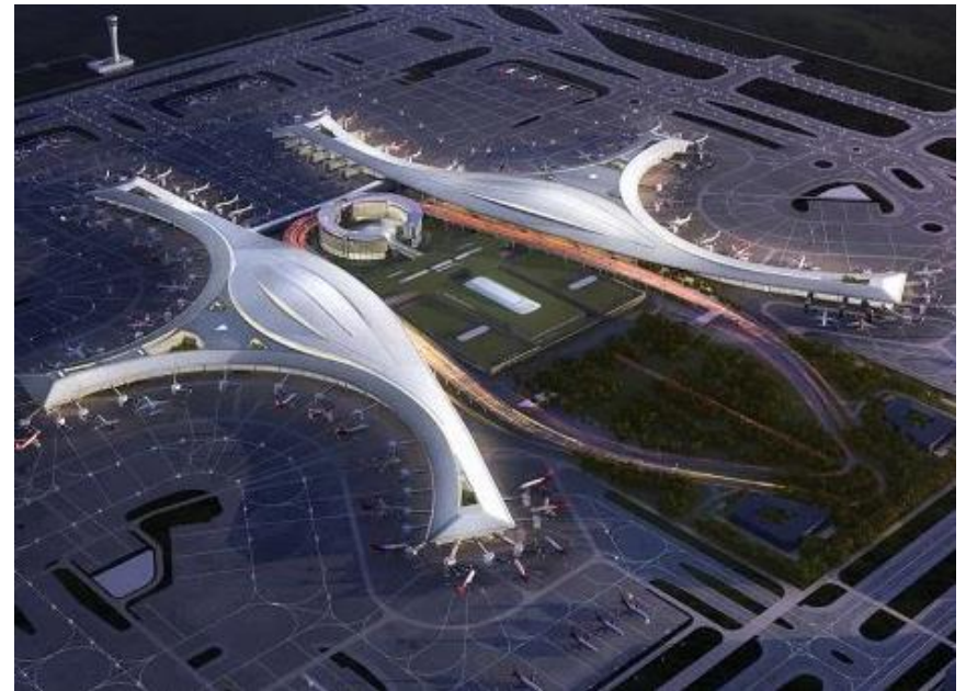
Chengdu Tianfu Airport, 210 gates
