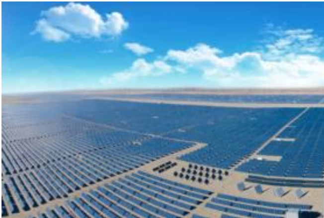
Golmud Solar Park 2.8 GW, world's largest
